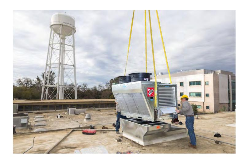
With the help of UC Davis facilities, Western Cooling Efficiency Center (WCEC) staff, and CalNEXT, we installed our field study unit: a CaptiveAire HP RTU!
