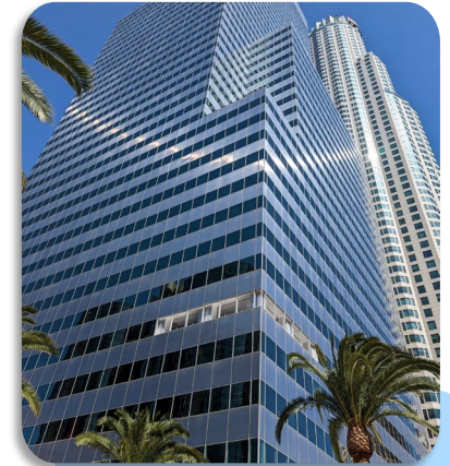
Commercial Building Efficiency Accelerator
